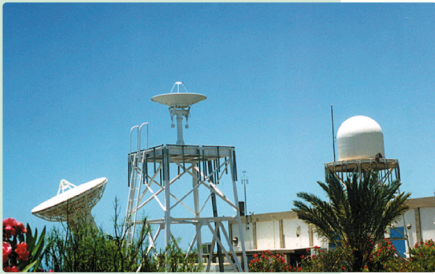
TTC operations antenna (15 m), MINISAT operations antenna (5 m) and COSPAS-SARSAT antenna (under dome).
