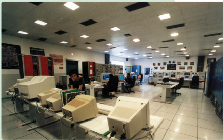
MER North operations room, devoted to earth resources operations with a 10-meter antenna.
