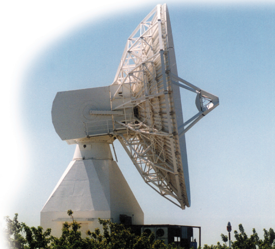
15 m antenna for TTC operations.
